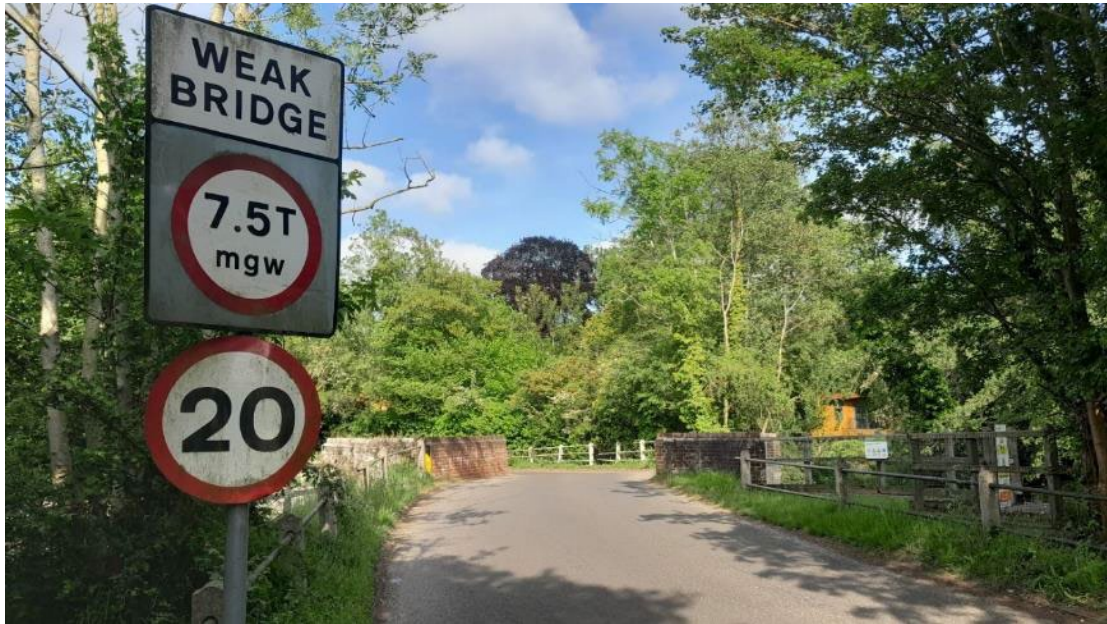
Figure 4-12 Costessey Mill Bridge, Costessey Lane
