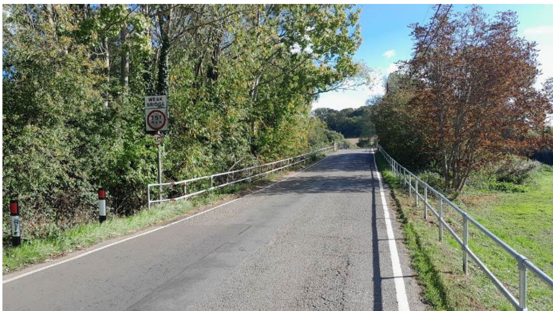
Figure 4-13 Ringland Road Bridge
