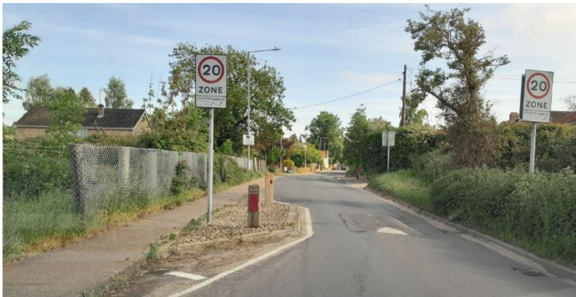
Figure 4-8 Traffic Calming Features at West End, Costessey
